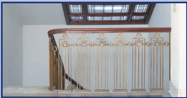
Decorative staircase metal work.
